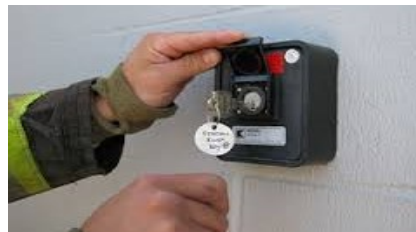
Store all building access keys in the Knox Box for emergency personnel use.
