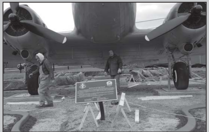
A cement curb and pad is being poured around static aircraft for better protection against the elements. The curbs will be completed this year and the pads will be poured weather permitting. After being poured, the curbs are covered with heating blankets until the cement cures. The aircraft are on loan from the National Museum United States Air Force. It is the base's responsibility to maintain display aircraft and to report on their condition annually. It is hoped the cement pads will protect the aircraft from damage. (Photos by Staff. Sgt Joseph McKee)
