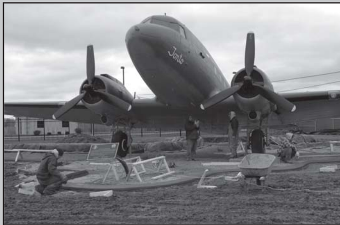
A cement curb and pad is being poured around static aircraft for better protection against the elements. The curbs will be completed this year and the pads will be poured weather permitting. After being poured, the curbs are covered with heating blankets until the cement cures. The aircraft are on loan from the National Museum United States Air Force. It is the base's responsibility to maintain display aircraft and to report on their condition annually. It is hoped the cement pads will protect the aircraft from damage. (Photos by Staff. Sgt Joseph McKee)
